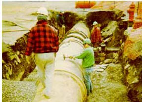
REPAIR CREW AT WORK
