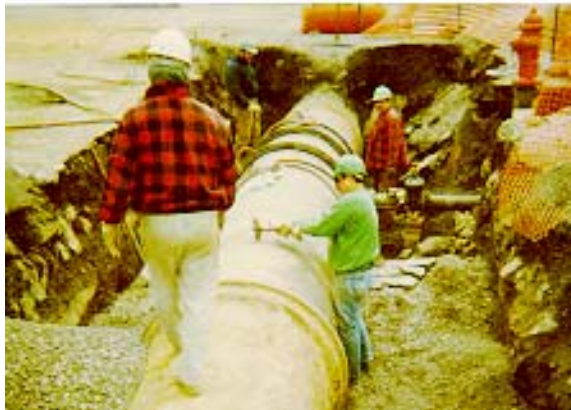
REPAIR CREW AT WORK
