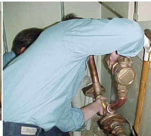
Placing resetter
