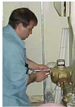
Unbolting flanges to
