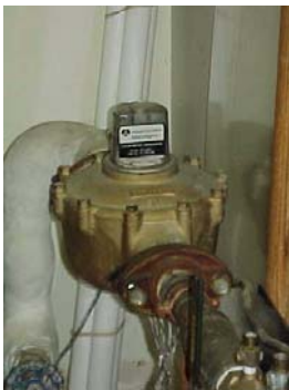
Old Flange meter on line before
