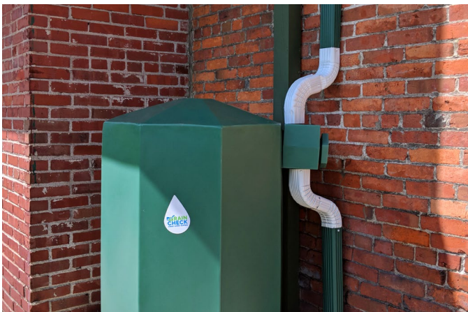
Rain barrel and downspout disconnection. Photo credit: Rain Check Buffalo.
